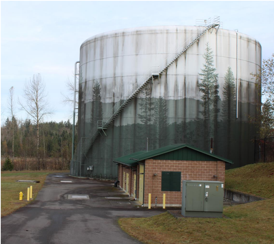
'4.3 Mil Gal Water Tank'
