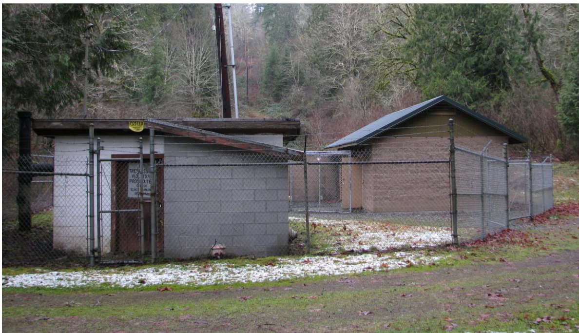
'Pump Station Building'
