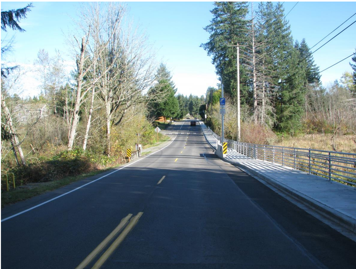
‘Roberts Dr. Walkway and Bridge Completion’
