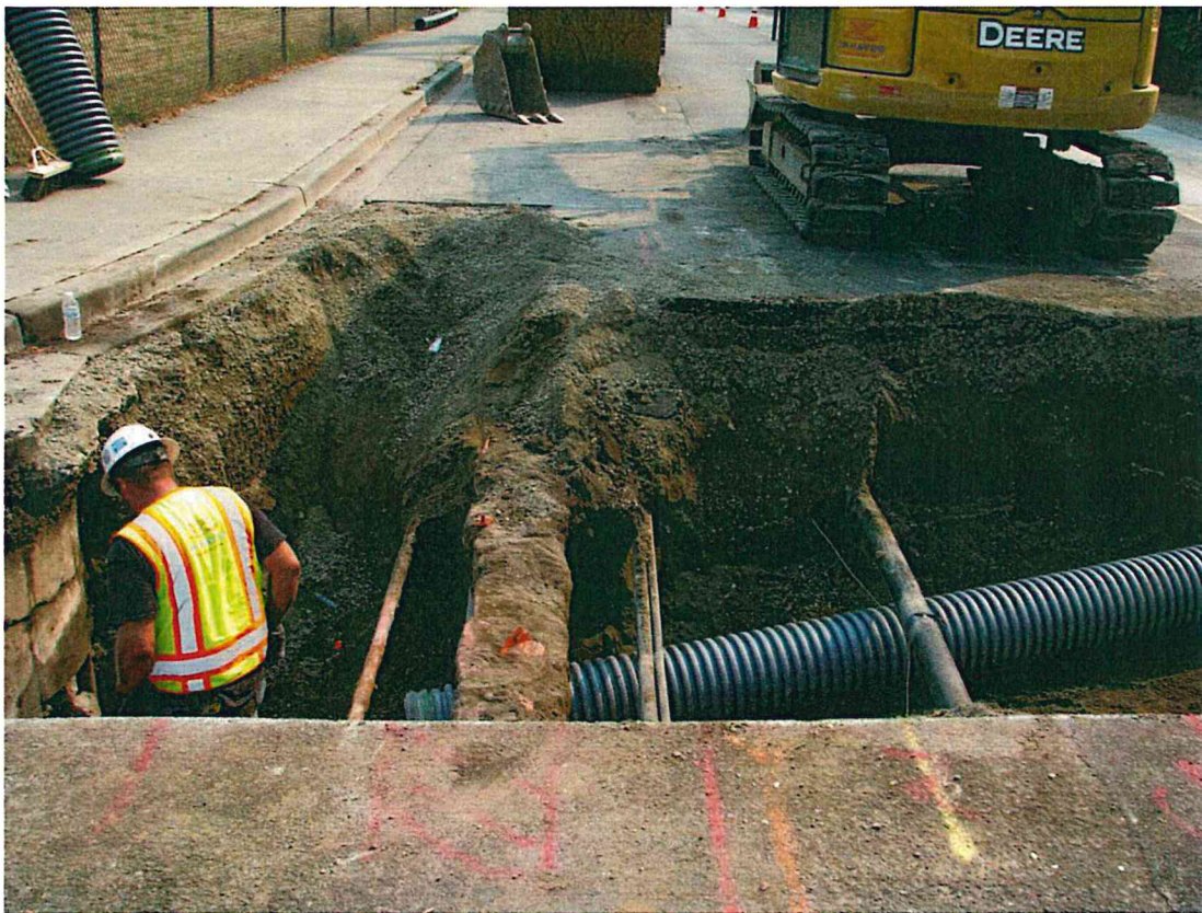
Installation of a stormwater pipe across Roberts Drive at Bruckners Way
