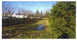
Example of a Bioswale to Help Filter Storm Water
