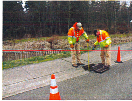
Catch Basin Inspection and Cleaning
